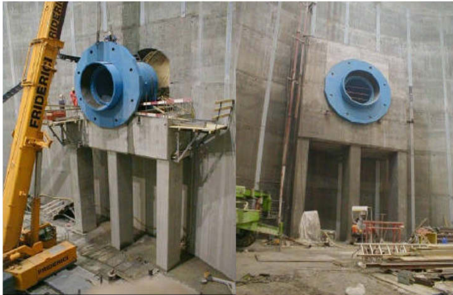
Fig. 2. TX1S Shielding installation in the underground cavern
